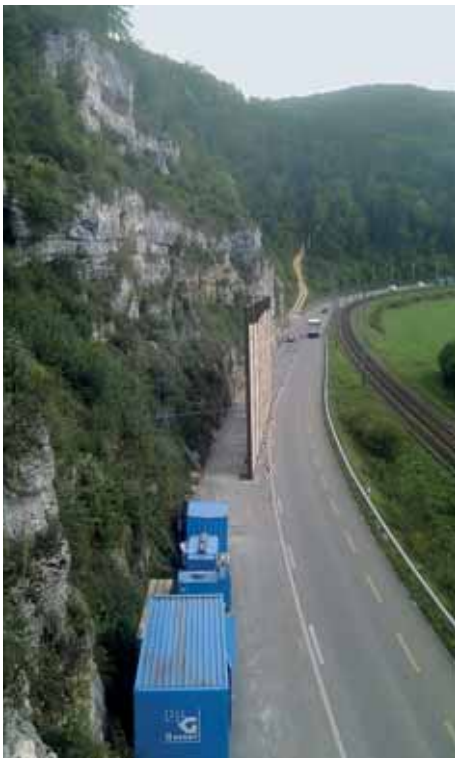
Bohlenwand 35 x 12 Meter.
