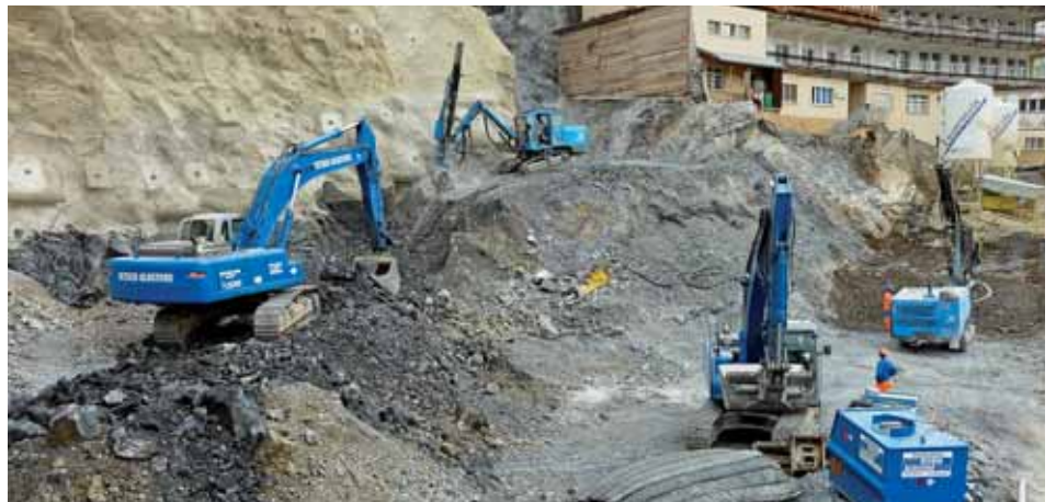
Baugrube Scarlett Sout.
