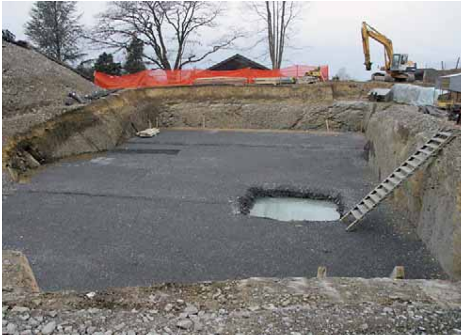
Baugrubenaushub 6'500m 3 .
