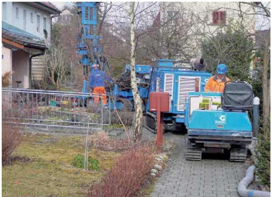
In Bohrposition an der Bettenstrasse in Winterthur.
